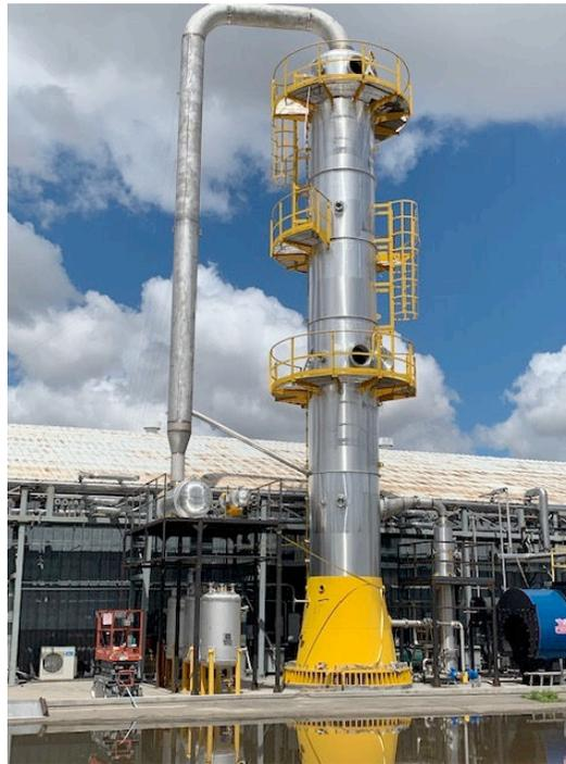
*A Biodiesel Decanter and Reboiler was installed adjacent to the 80-foot tall biodiesel distillation column that will refine-out any remaining micro-particulates.*
